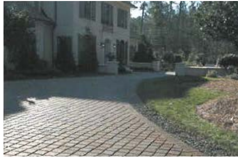
Innovative permeable pavement creates an upscale look for driveways; it also helps builders comply with local stormwater regulations.
