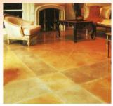
Stamped and Textured Concrete—using this method, semi-hardened fresh concrete is stamped with special tools that make plain concrete mimicmaterials such as slate, stone, or brick. With advancements in stamping tools and coloring methods, it's almost impossible to distinguish between natural materials and decorative.
