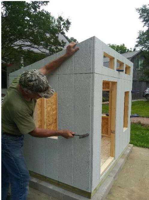
Figure 33. Attach side wall sheathing to front wall frame
