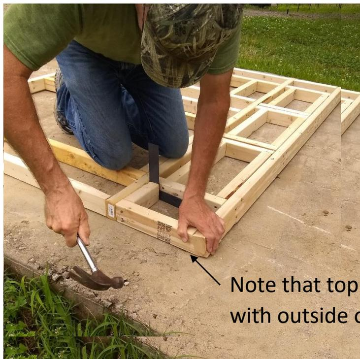
Figure 26. Use blocking (with shims) while toenailing
