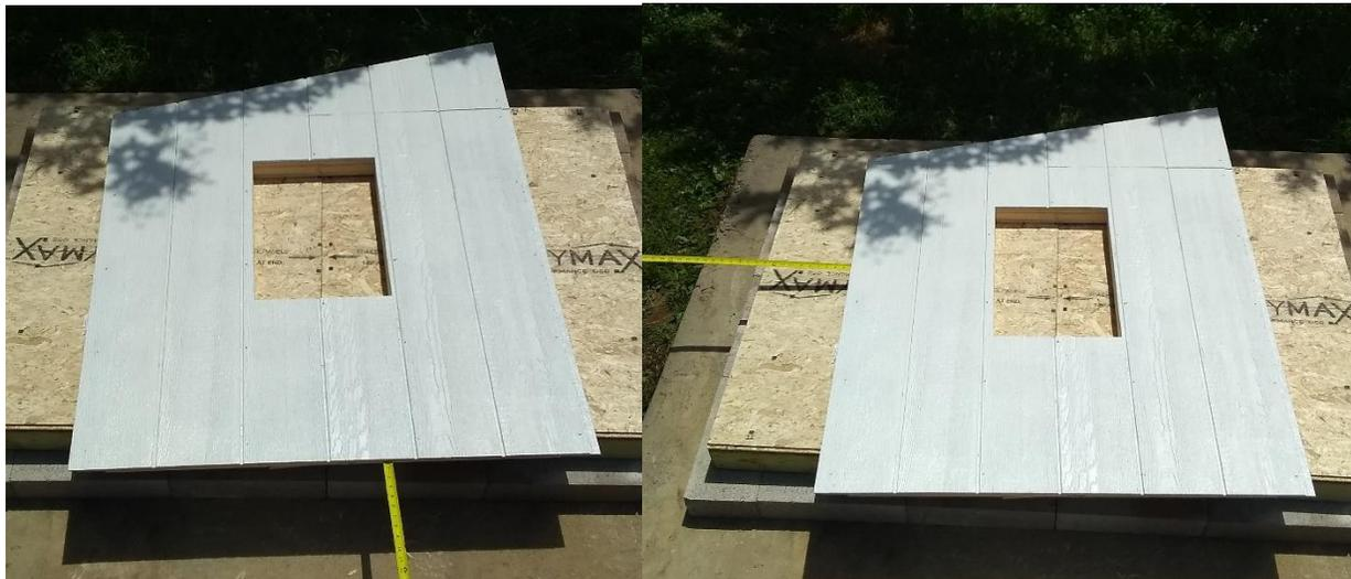
Figure 29. Align siding with the required overhang
