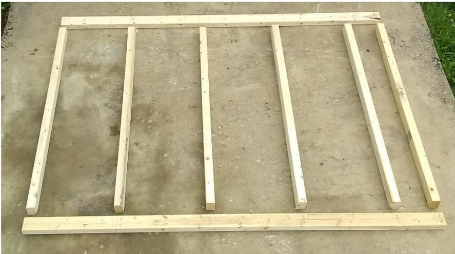
Figure 7b. Photograph of back wall framing prepared for assembly
