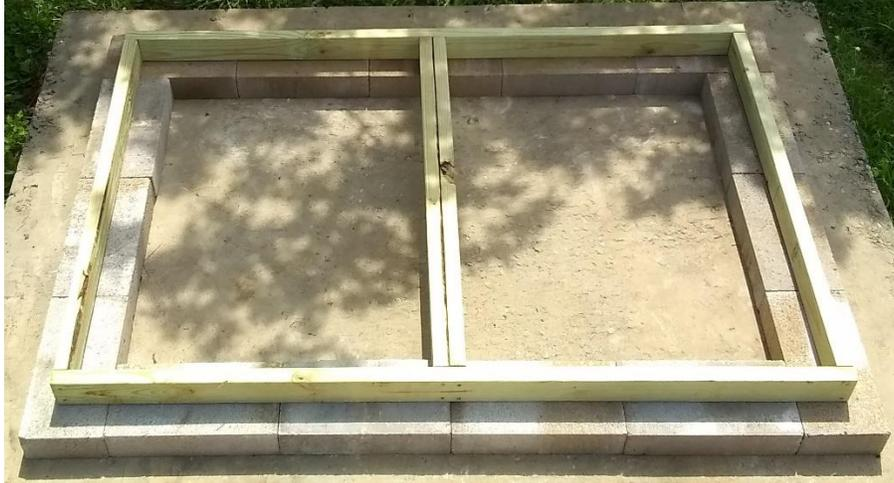
Figure 19. Photograph of floor framing placed on foundation.
