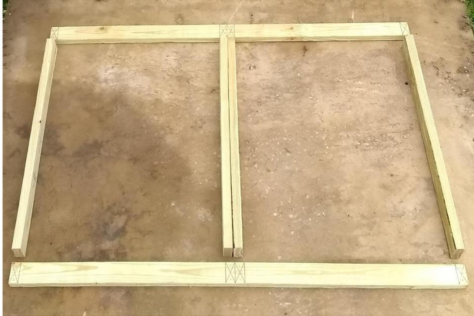
Figure 4. Photograph of Floor framing prepared for assembly
