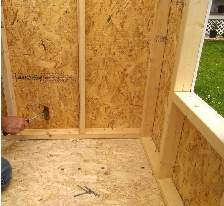
Figure 31. Nail walls to floor
