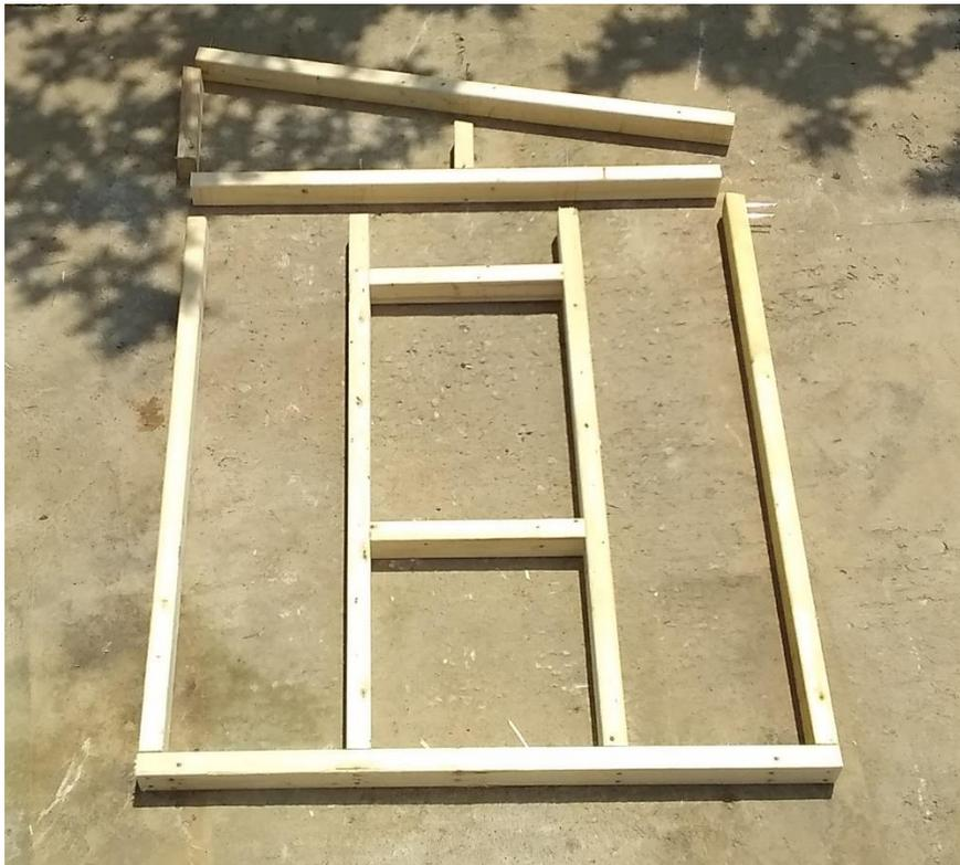
Figure 28. Right wall framing assembly photograph
