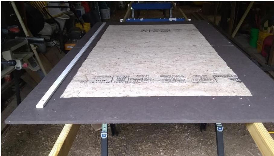
Figure 34. Trim attached to underside of roof
