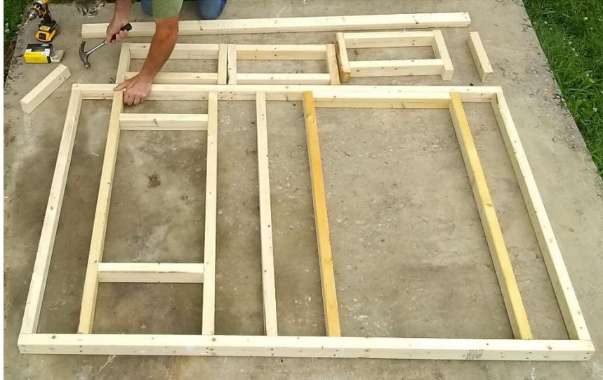
Figure 25. Toenailing is required in places
