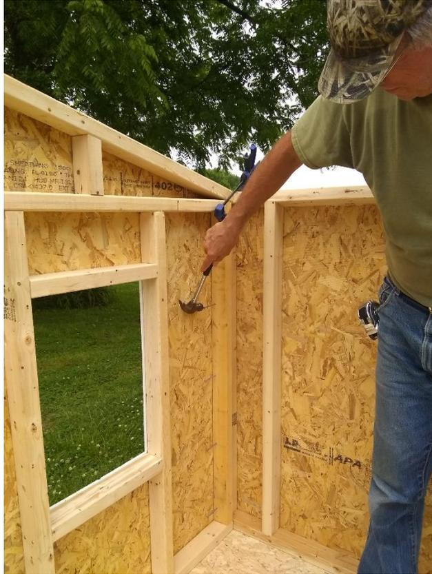
Figure 32. Finish driving nails to secure walls
