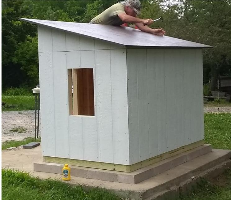
Figure 36. Nail roof to walls
