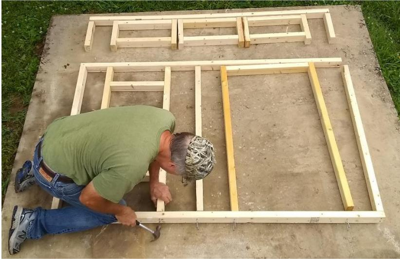
Figure 24. Complete the bottom 4-foot frame
