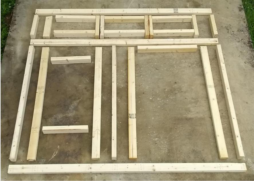
Figure 7a. Photograph of front wall framing prepared for assembly
