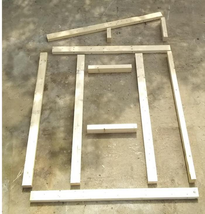
Figure 7c. Photograph of left wall framing prepared for assembly
