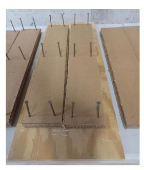
Figure 7. Start nails in deck boards
