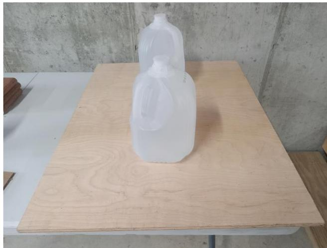
Figure 5. Weight the deck boards to dry
