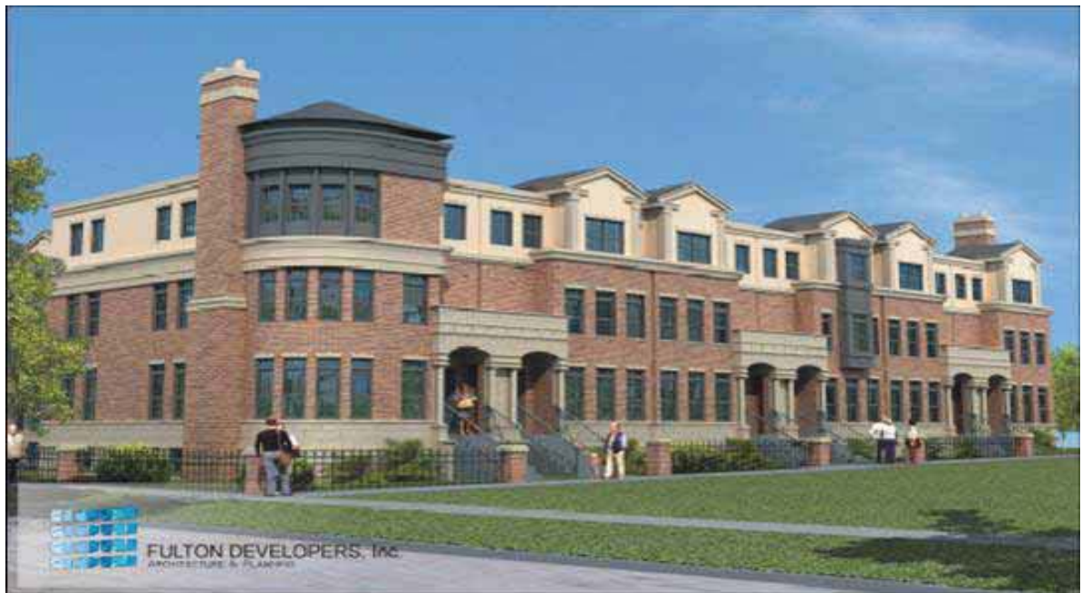
Laurel Court is a new 15-unit development that includes two affordable units.
