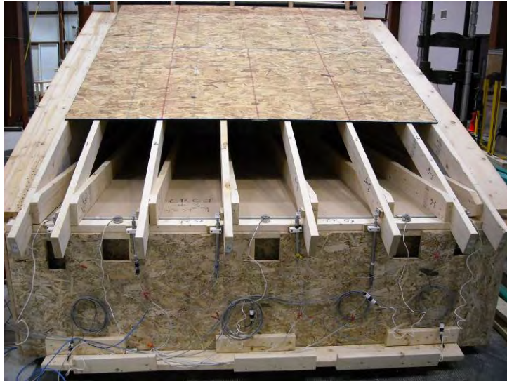
Figure 4 – Uplift set-up instrumentation (OSB panel is not attached to show connections and instrumentation)
