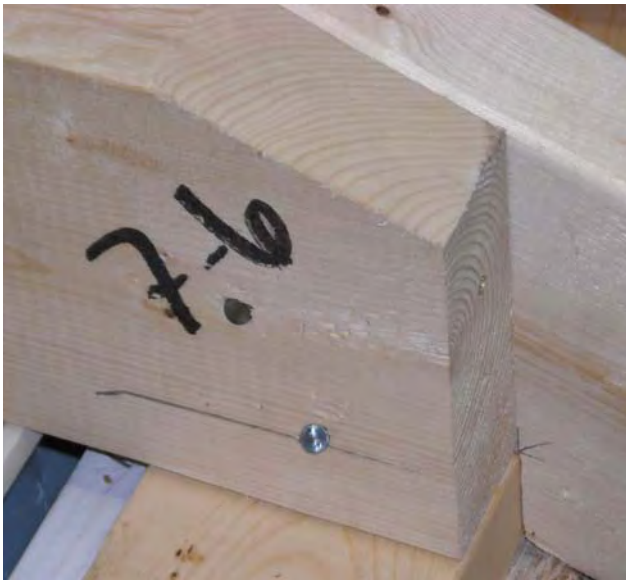
Figure 8 – Installation of toe-nails
