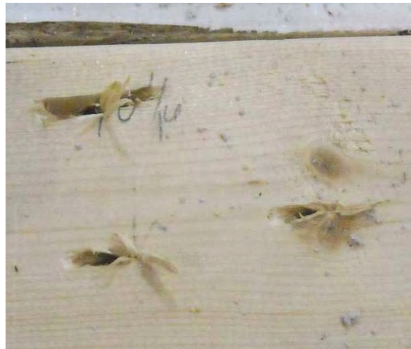
Figure 21 – Local tearing/crushing of top plate associated with withdrawal failure mode
