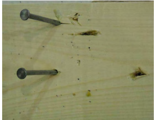
Figure 16 – 16d nails in plate after pull-through failure
