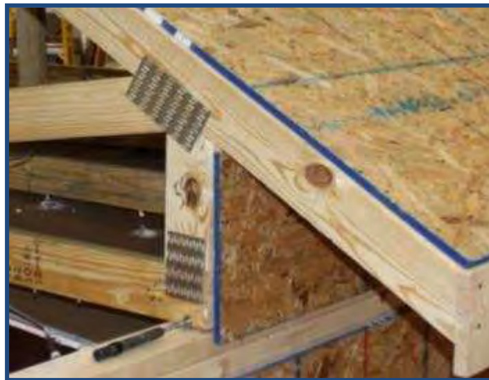
Figure 18 – Truss rotation of Specimen E at failure (Truss 5)
