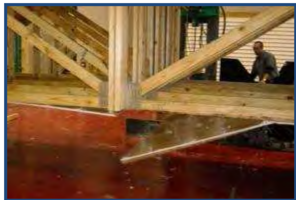
Figure 12 – Complete failure of gypsum fasteners (Specimen A)
