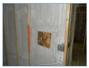
Figure 5. Sensor After Foam Flash and Before Insulation
