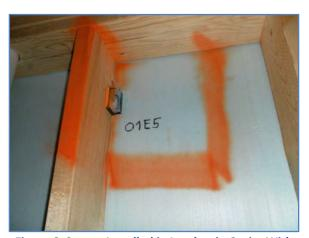
Figure 6. Sensor Installed in Lumber in Cavity With Only Foam Sheathing
