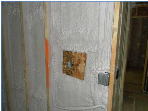
**Figure 5. Sensor After Foam Flash and Before Insulation**
