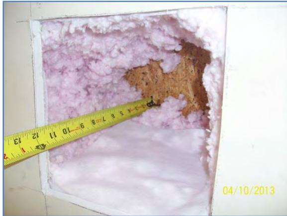
**Figure 53. Insulation Removed from R-46 Wall for Observation**
