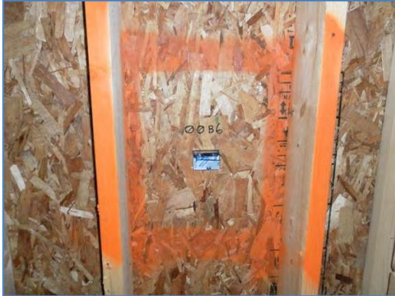
**Figure 3. Sensor Installed in OSB Sheathing That Will be Foamed Over in This Test House**
