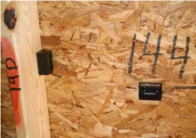
Figure 5. Sensors installed in the oriented strand board and stud
