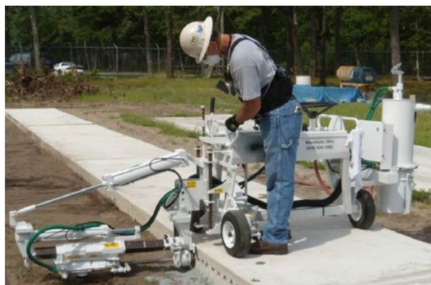
Worker drilling horizontal holes in concrete slab with a dowel drilling rig. The shroud surrounds the drill steel where it enters the concrete and the dust collector is the canister on the right. Worker is wearing respiratory protection.
