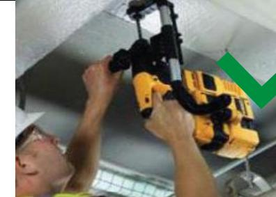
Worker drilling into concrete with a rotary hammer equipped with shroud and dust collection system.
