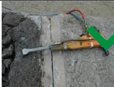
Jackhammer equipped with water spray delivery system.
