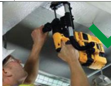
Worker drilling into concrete with a rotary hammer equipped with shroud and dust collection system.
