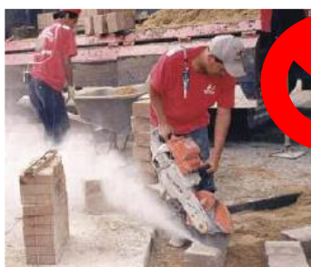
Worker using handheld masonry saw without any dust controls.
