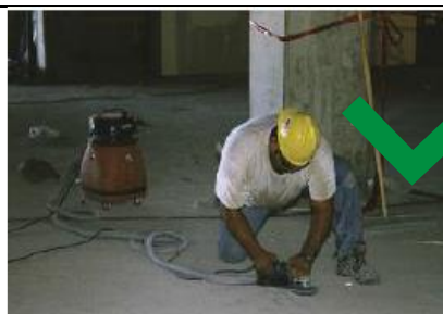
Worker using a grinder on concrete with a dust collection system.
