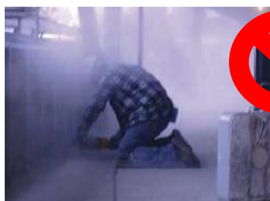
Worker using grinder on concrete without any dust controls.
