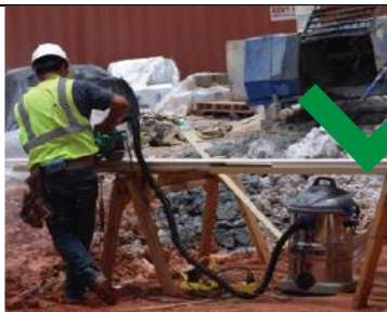
Worker cutting fiber cement with a handheld saw and dust collection system.
