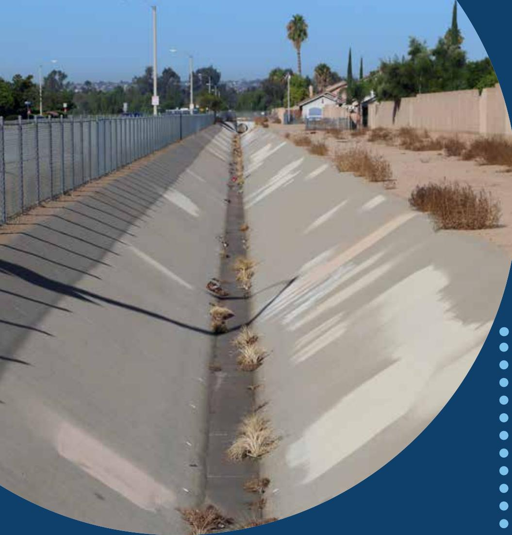
*Traditional drainage infrastructure uses pipes and concrete to move water away from sites as quickly as possible. Today stormwater requirements often ask developers to infiltrate or capture water on-site.*
