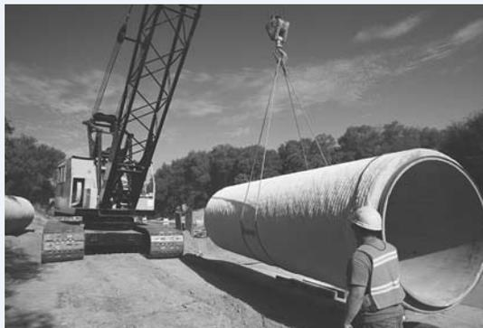
constructing an effluent disposal system. In most cases, discharge is directed into suitable soils where additional treatment takes place and the groundwater table is ultimately recharged.
