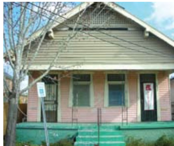
This house will be remodeled by National Green Building Conference and 50+ Housing Symposium attendees.
