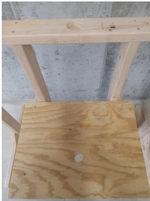
Figure 3. Holes for vent pipe and sink tail piece
