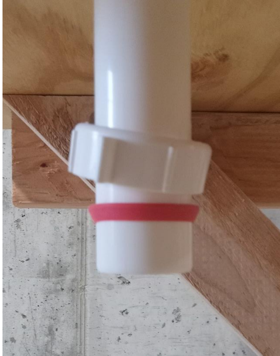
Figure 9. Place seal on tailpiece
