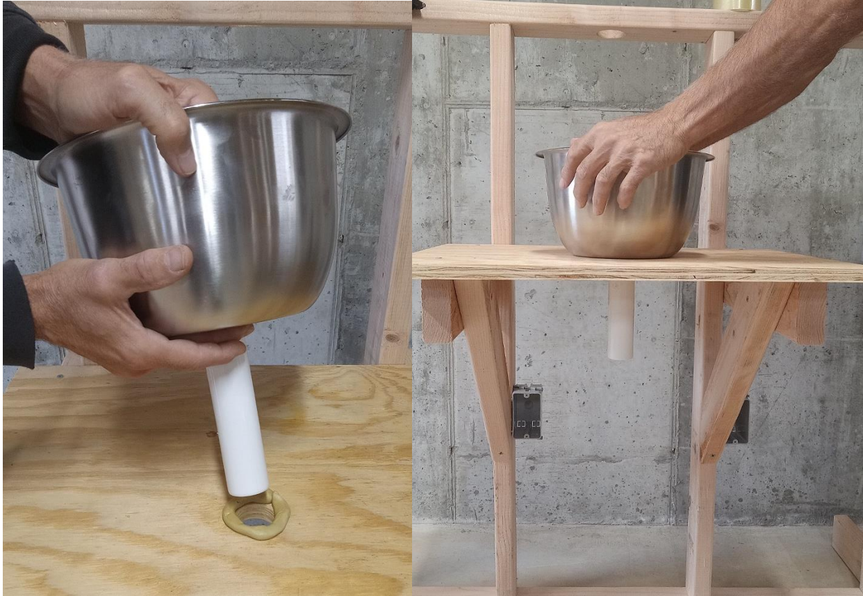
Figure 8. Install the sink w/tailpiece
