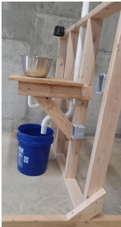
Figure 1. Completed Plumbing Wall
