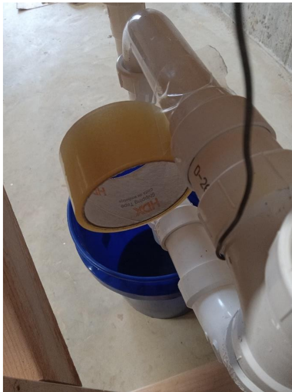
Figure 10. Tape the slip joint to minimize leakage
