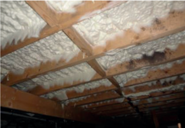
FIGURE 17. Installation of SPF below the subfloor allows complete access to the band joist and sill plate for inspection.
