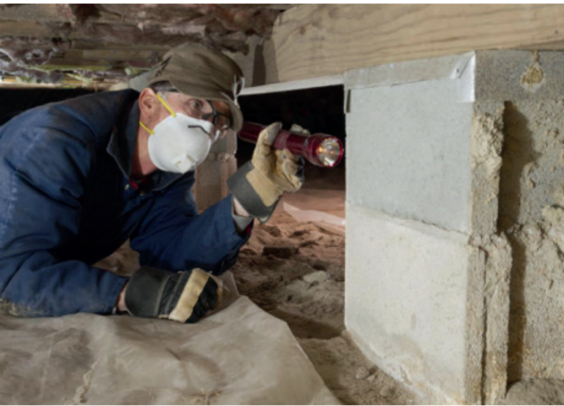
FIGURE 3. Visual termite inspection
