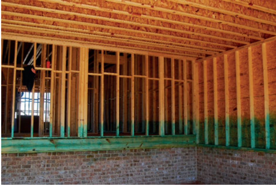
FIGURE 6. Borate treatment of select structural wood components
